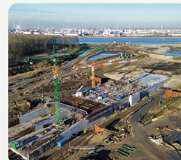
Drone image of Oosterweel construction site
