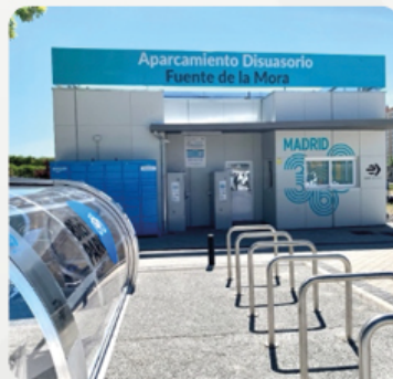
Park & Ride facility in Fuente de la Mora, in Madrid (Spain)
