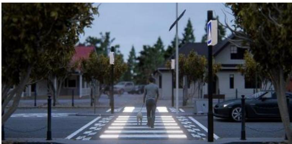
Figure 55. Intelligent crosswalk system (Funchal, Portugal).
