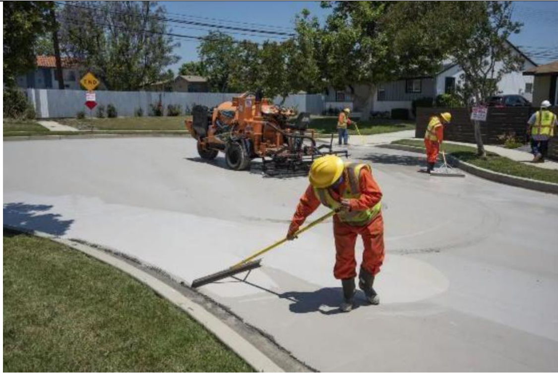
Figure 67. Reflective asphalt coatings (Los Angeles, USA).
