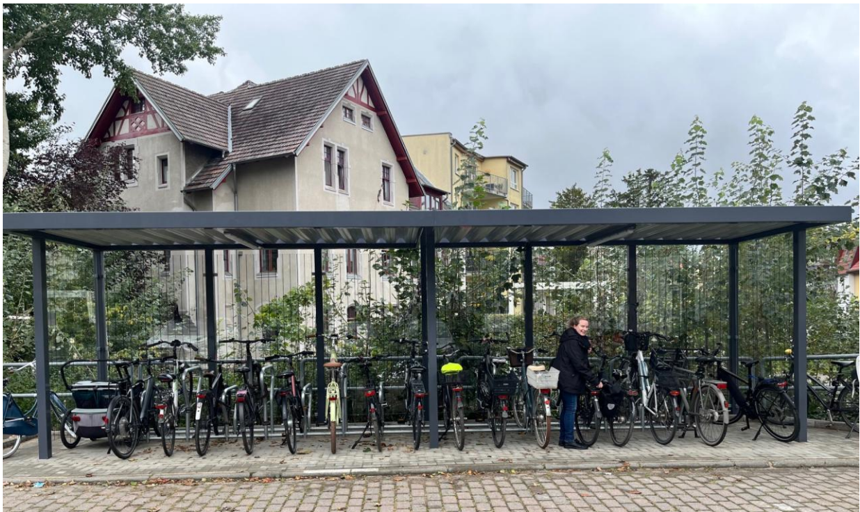
Figure 1. Permanent weather-protected bicycle parking facility. Author: Stephan Braun
